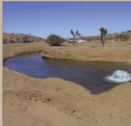
Groundwater recharge basin
