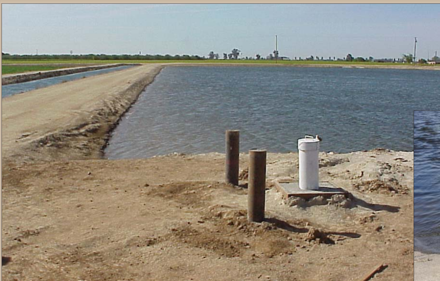
Recharge basin monitoring well
