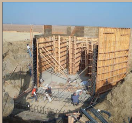
Framework for pumping plant and basin
