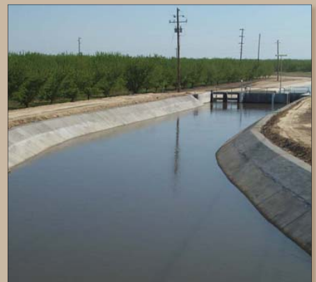
New lining raised the canal to increase capacity
