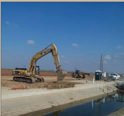
Excavating for turn out and pump basin
