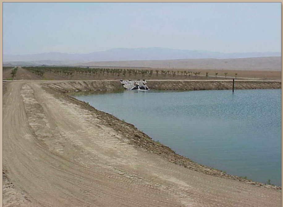
A partial view of the pilot recharge basin with the inlet shown in the background.
