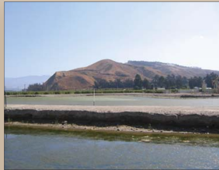
Saticoy spreading grounds recharge facility
