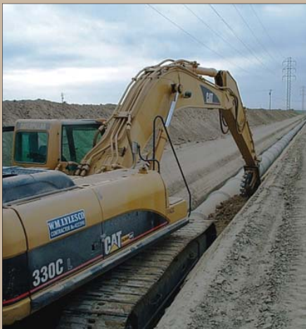
Preparing trench for pipe
