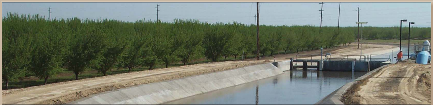
Semitropic canal lining height augmentation
